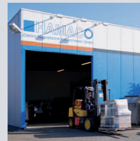
Loading of the cabin components for transport
